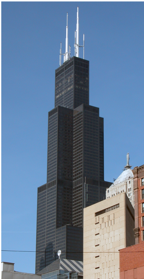
Figure 2. Diagonal bracing system of the John Hancock Tower in Chicago, Illinois. (top images) In addition to reinforcing the tubular steel frame, the diagonals provided for alternate load paths. 6 The Willis Tower (bottom images) uses a bundled tube system to resist wind loading of the cantilevered form. This structural arrangement does not allow significant areas for open office planning, particularly towards the top of the tower. Stepping back the top decreases wind resistance. 7
